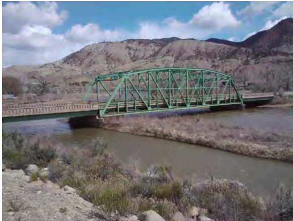
Dotsero Bridge, Eagle County, 2013
