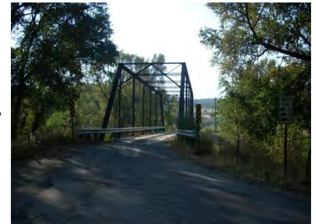
Paonia Bridge, 1911 Medium Priority
