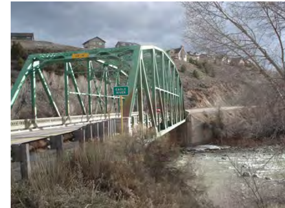
Eagle River Bridge, Eagle County, 2012
