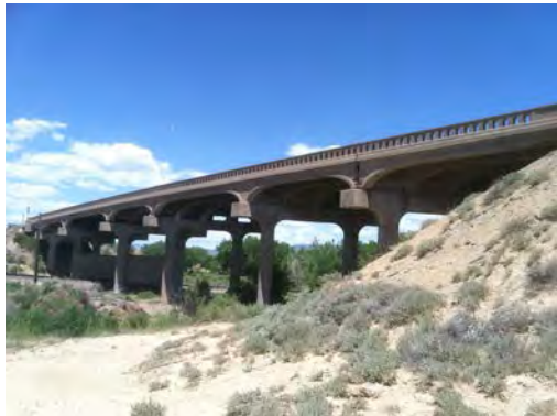
Rio Grande Railroad Viaduct, 2015
