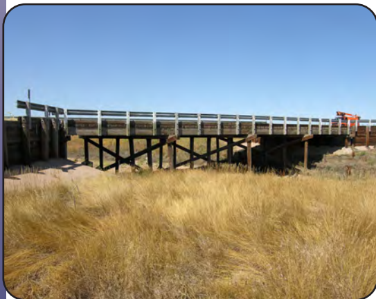
Image 18. SH 61 over Surveyor Creek in Washington County (D-25-E)
