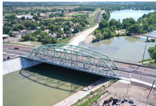
Santa Fe Avenue Bridge, Pueblo County, Rehab
