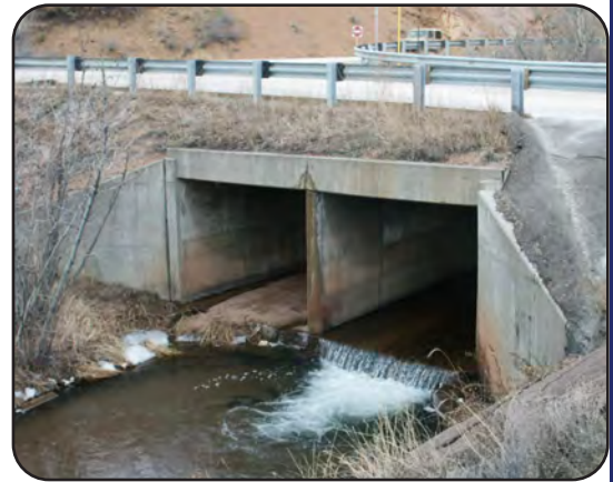
Image 17. US 24 Service Rd over Fountain Creek in El Paso County (I-17-X)
