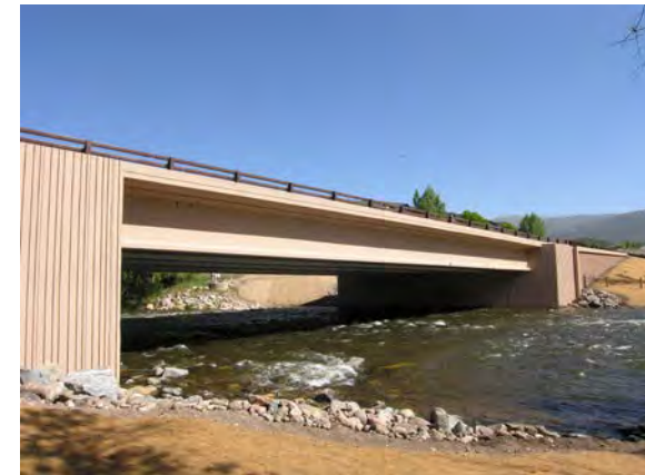
Structure F-09-AS (Eagle River)
