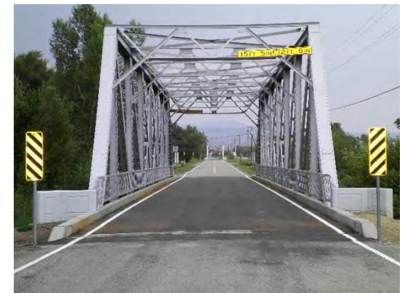
Twin Gunnison River Bridges, Gunnison County, Rehab
