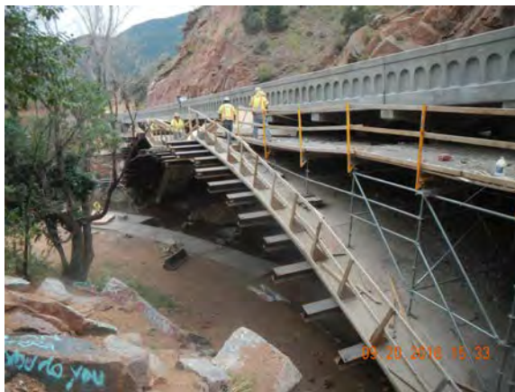
Rainbow Falls, El Paso County, Rehab
